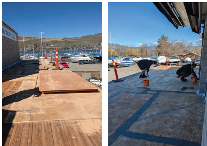
Deck Under Construction Hard at Work on the New Deck
