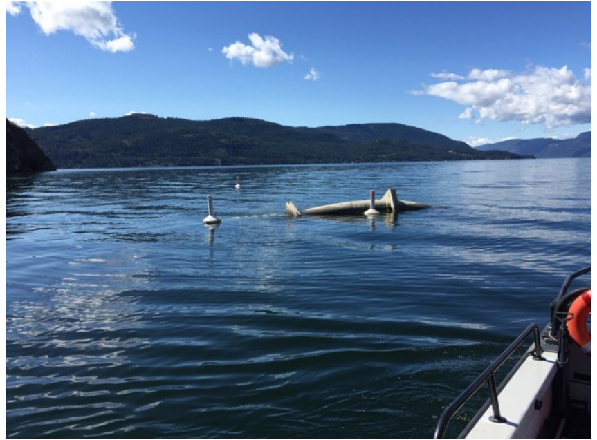
Even the City of Vernon needed Station 101's help when an outflow pipe surfaced.
