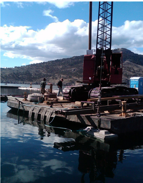
Burton Marine prepares to drop one of the 2000KG anchors that will hold the C dock extension in place.. (Photo's by Dan Irvine)
