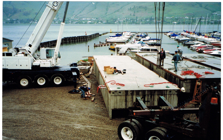
Building concrete breakwater 1988
